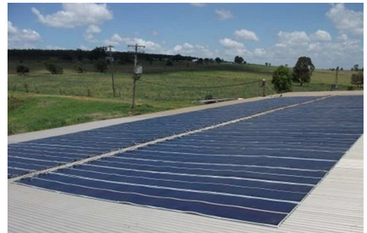
Above: The flexible, lightweight silicon cells are unpacked, ready for installation. Below: The SKYShades solar cell installation will power machinery in the Crumpton's peanut processing shed as well as feed electricity back into the grid.
